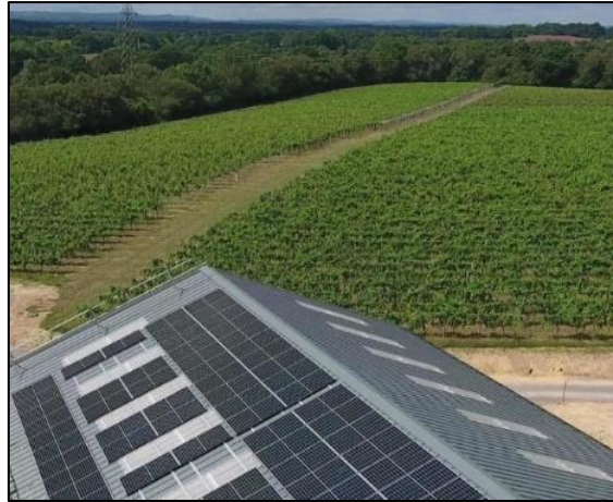
Figure 5: 60kW of P.V. Array at Bolney Wine Estate (Community Solar Energy Projects, 2019)
